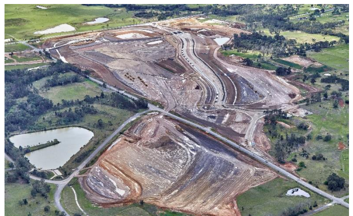
Early earthworks site, October 2019
