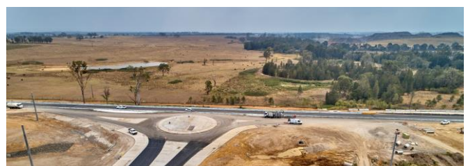
New Elizabeth Drive Roundabout under construction December 2019
