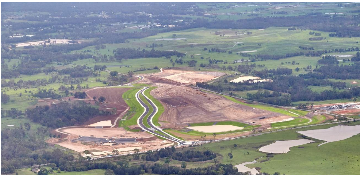
The new Elizabeth Drive and Badgerys Creek Road intersection
