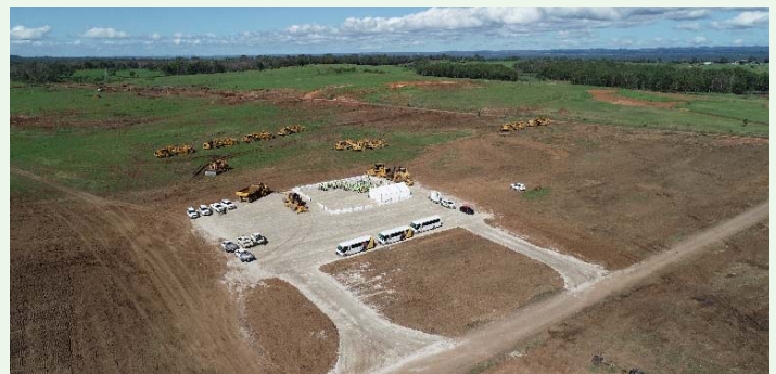
Bulk earthworks media event March 2020
