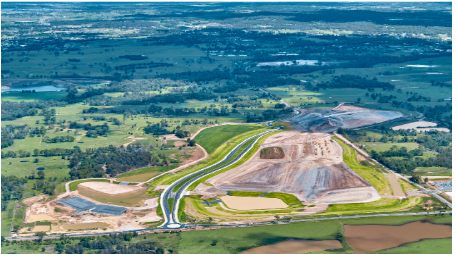
An aerial view of the Early earthworks site in March 2020
