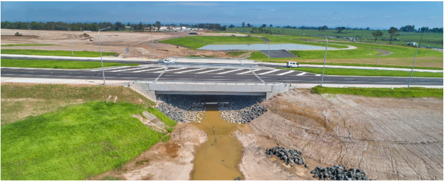
The new Badgerys Creek Road bridge in February 2020
